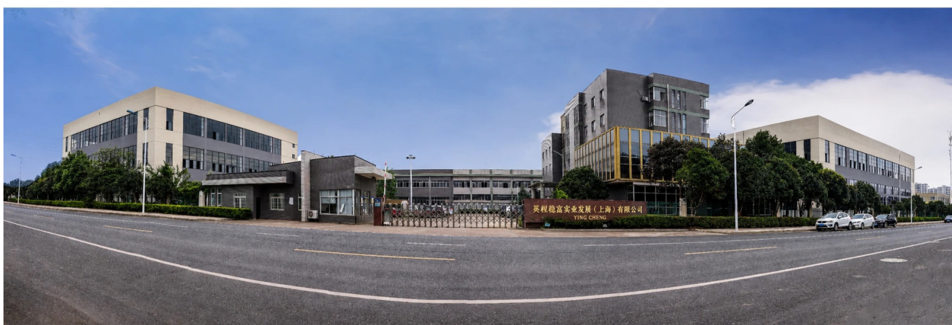
Factory exterior · branding presentation
